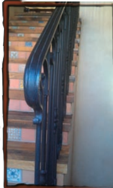
3/4" x 1 1/2" Chisel cut with lamb's tongue
